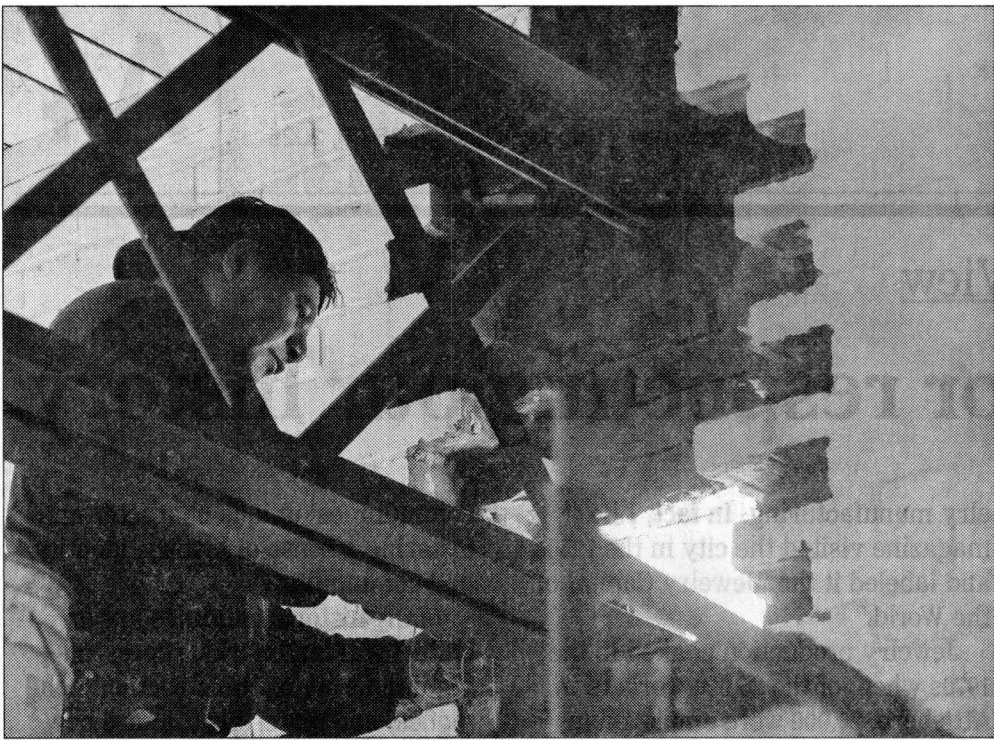
PHOTOS BY PAUL CONNORS / THE SUN CHRONICLE Mason Emilio Cruz recently repairs brickwork on one of the storage buildings that's a part of the historic Sadler Mill complex in South Attleboro.
